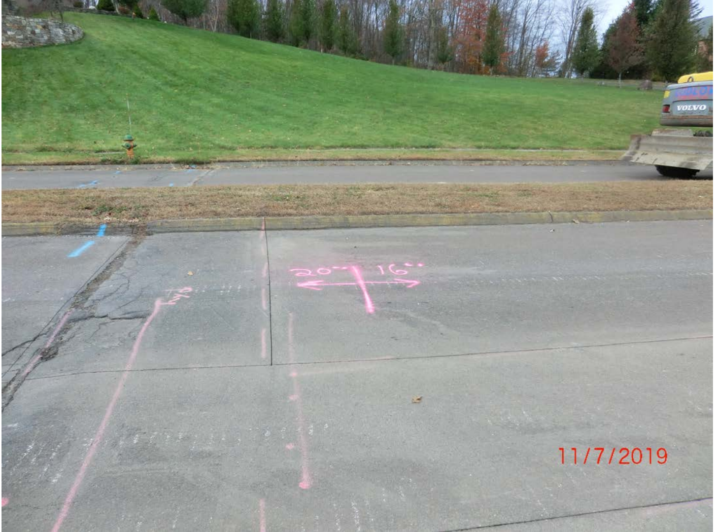
Figure 8 – Mark out for cross over from 16” to 20” DIP. Will not likely be reached by end of week given issues with solid bedrock and a number of utility crossings between current location and here.
