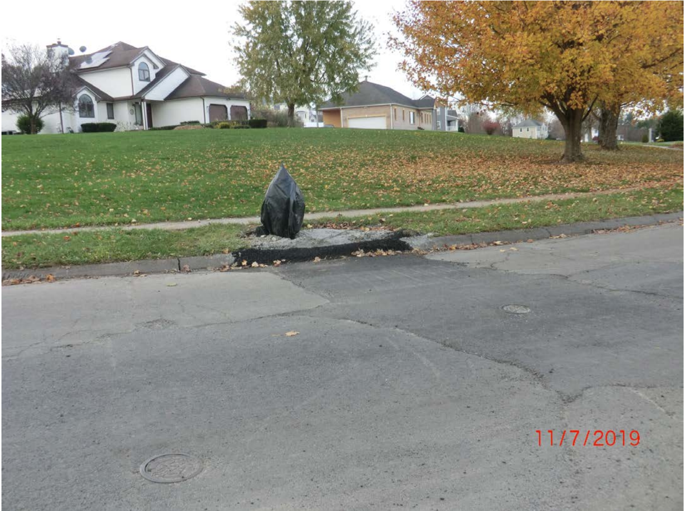
Figure 3 – Facing northwest. New hydrant installation on Talcott Ridge Dr. at intersection with upper Watch Hill Dr. (not shown but located to the left of this shot).
