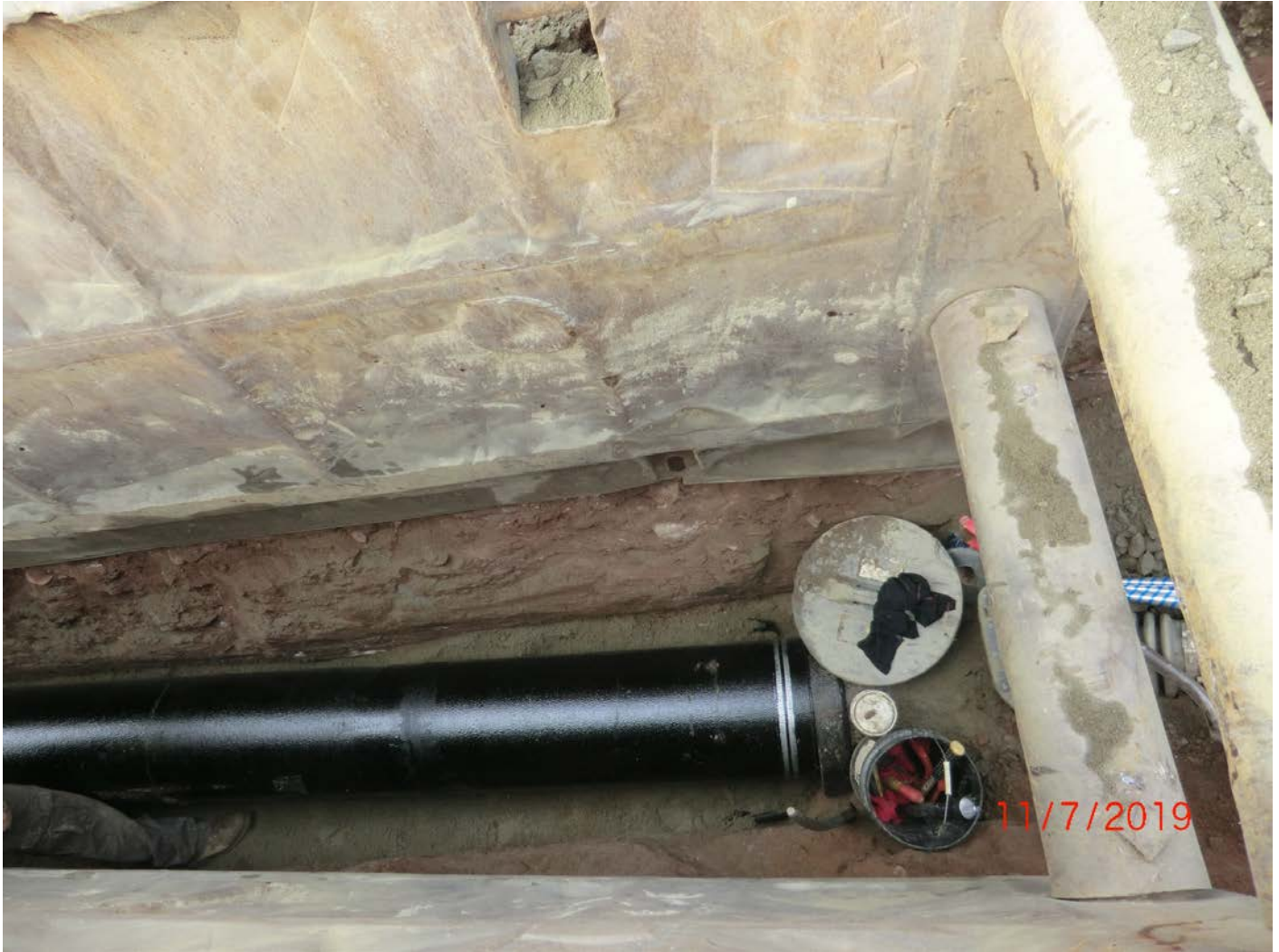
Figure 6 – Setting pipe. Note position of silver rings on pipe. This indicates that the pipe has not yet been fully seated into bell to right.
