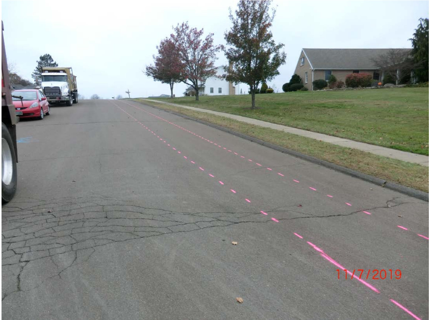
Figure 13 – Road cut mark out for upper Watch Hill Drive replacement hydrant 8” DI line. Photo taken facing west.
