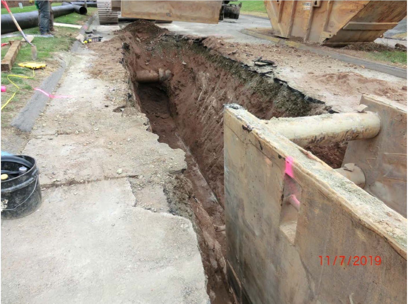
Figure 15 – Facing south, water service line can be seen just left of the end of the trench box and in the distance, just beyond the end if the final stick of pipe (not yet placed in trench) is the culvert drain line.
