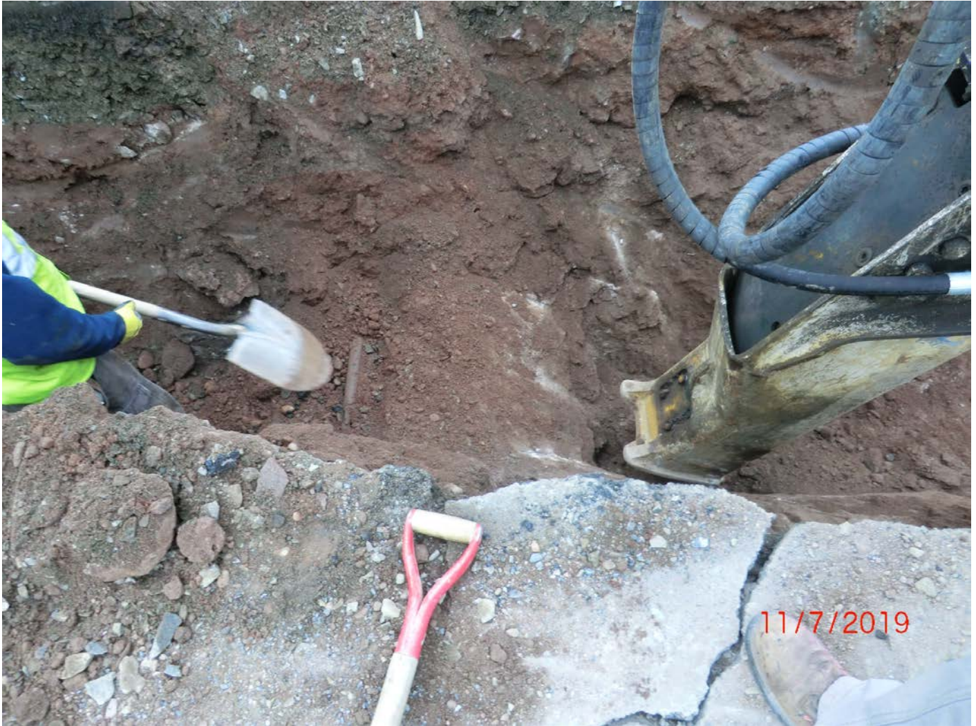
Figure 11 – Hammering rock out from under water service line (seen just in front of shovel).
