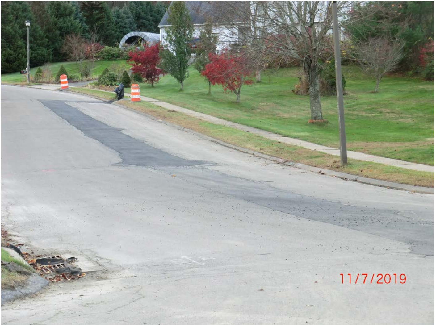
Figure 1 – Facing south-southwest. 8”-DI pipeline up lower Watch Hill Drive to new hydrant.
