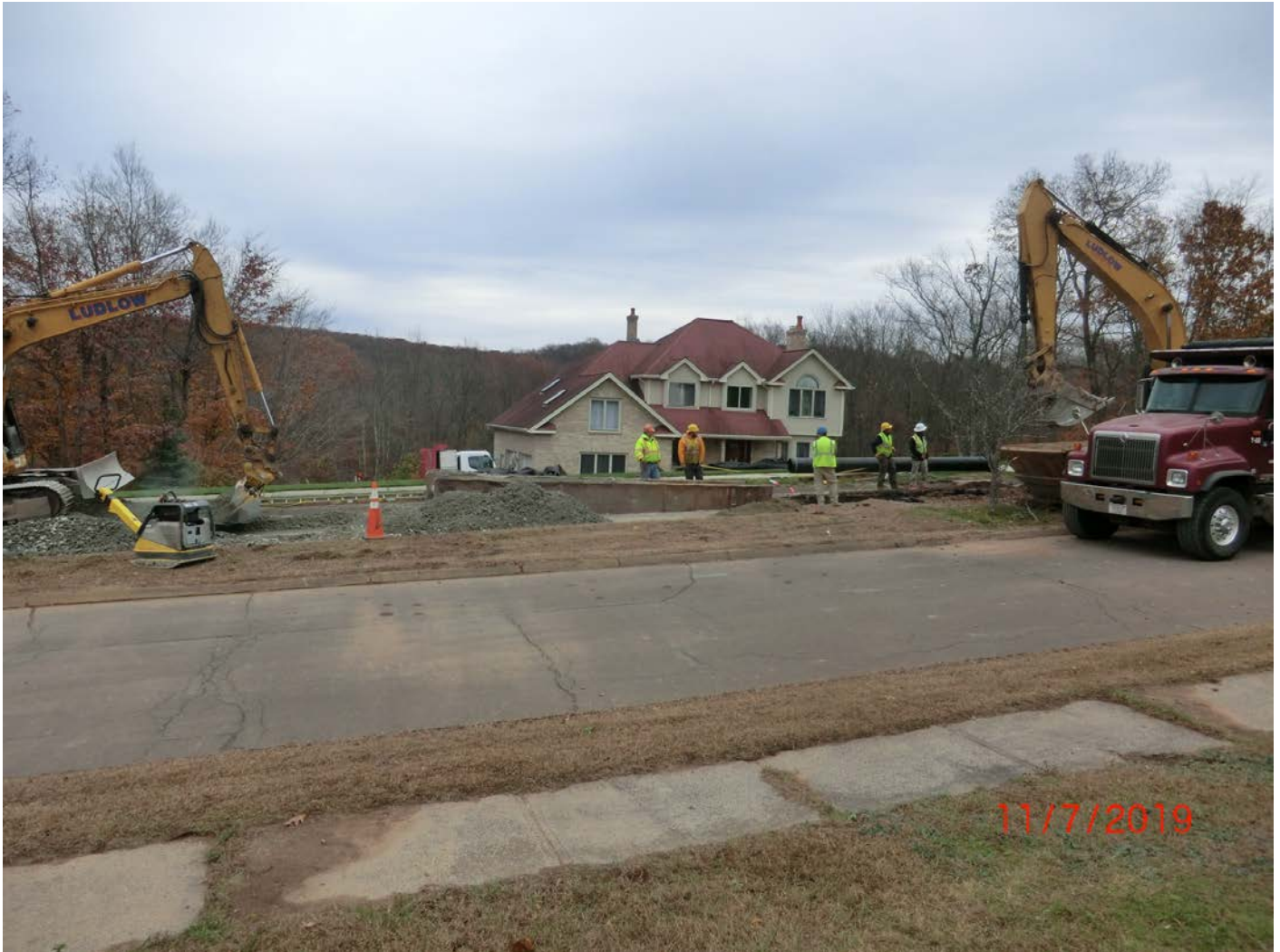
Figure 14 – Broad perspective of today's work. Photo taken facing east.
