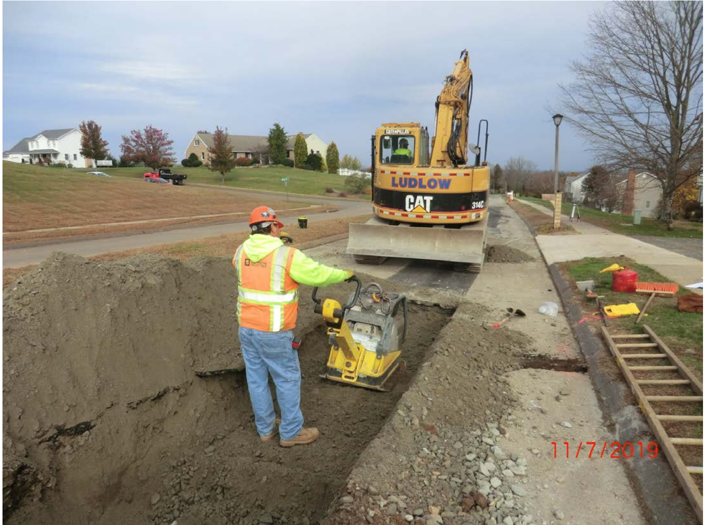
Figure 7 – Facing north. Lift compaction with Wacker plate compactor. Upper Watch Hill Drive seen in background to left.
