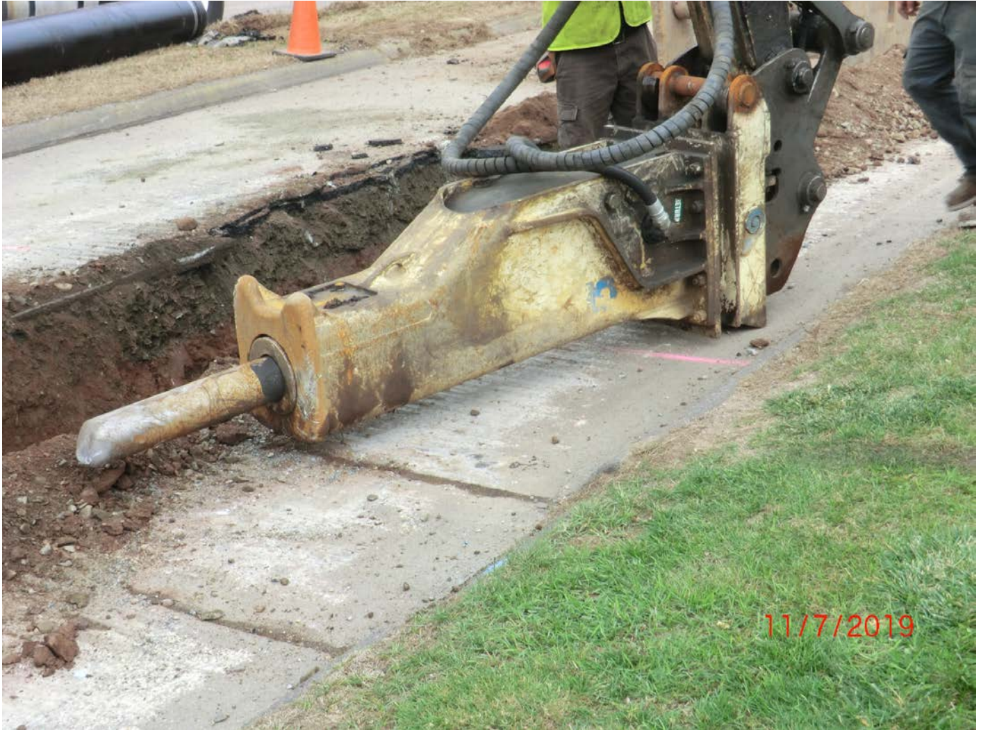
Figure 9 – Ram hammer used to break up bedrock for removal. Process often requires a widening of the trench to be able excavate the width to insert the 16” DI.
