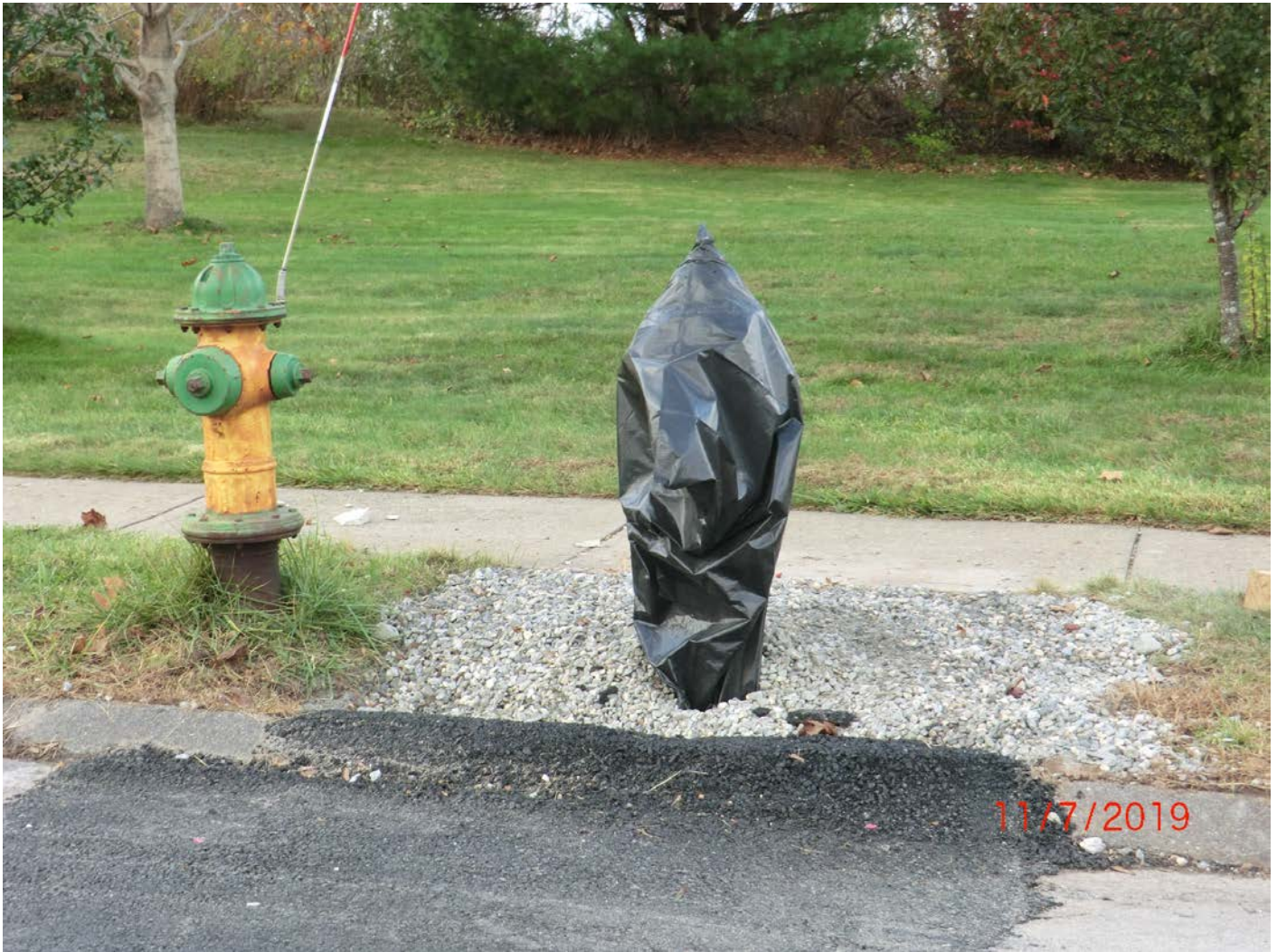
Figure 2 – Facing south – New hydrant installation on lower Watch Hill Drive.
