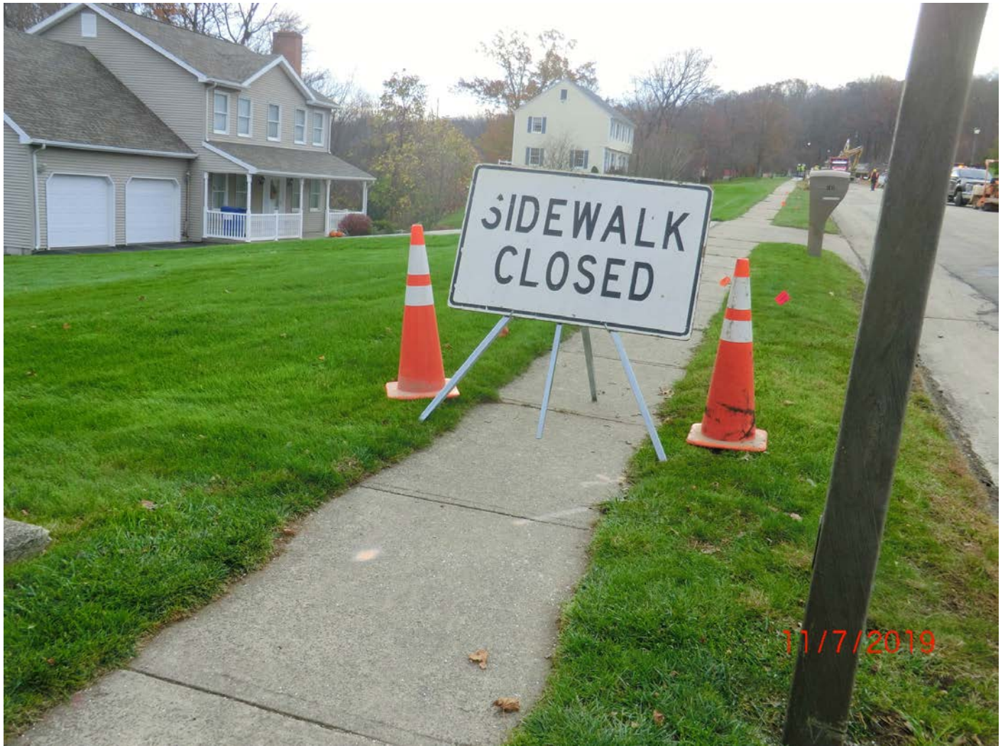
Figure 5 – Sidewalk closure sign. Photo taken facing south.
