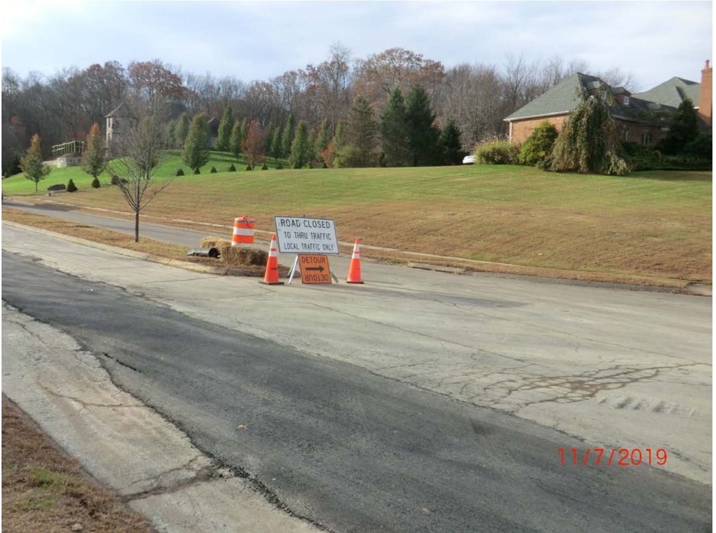
Figure 4 – Facing southwest, road closure sign. Upper Watch Hill Drive to the right of this shot.
