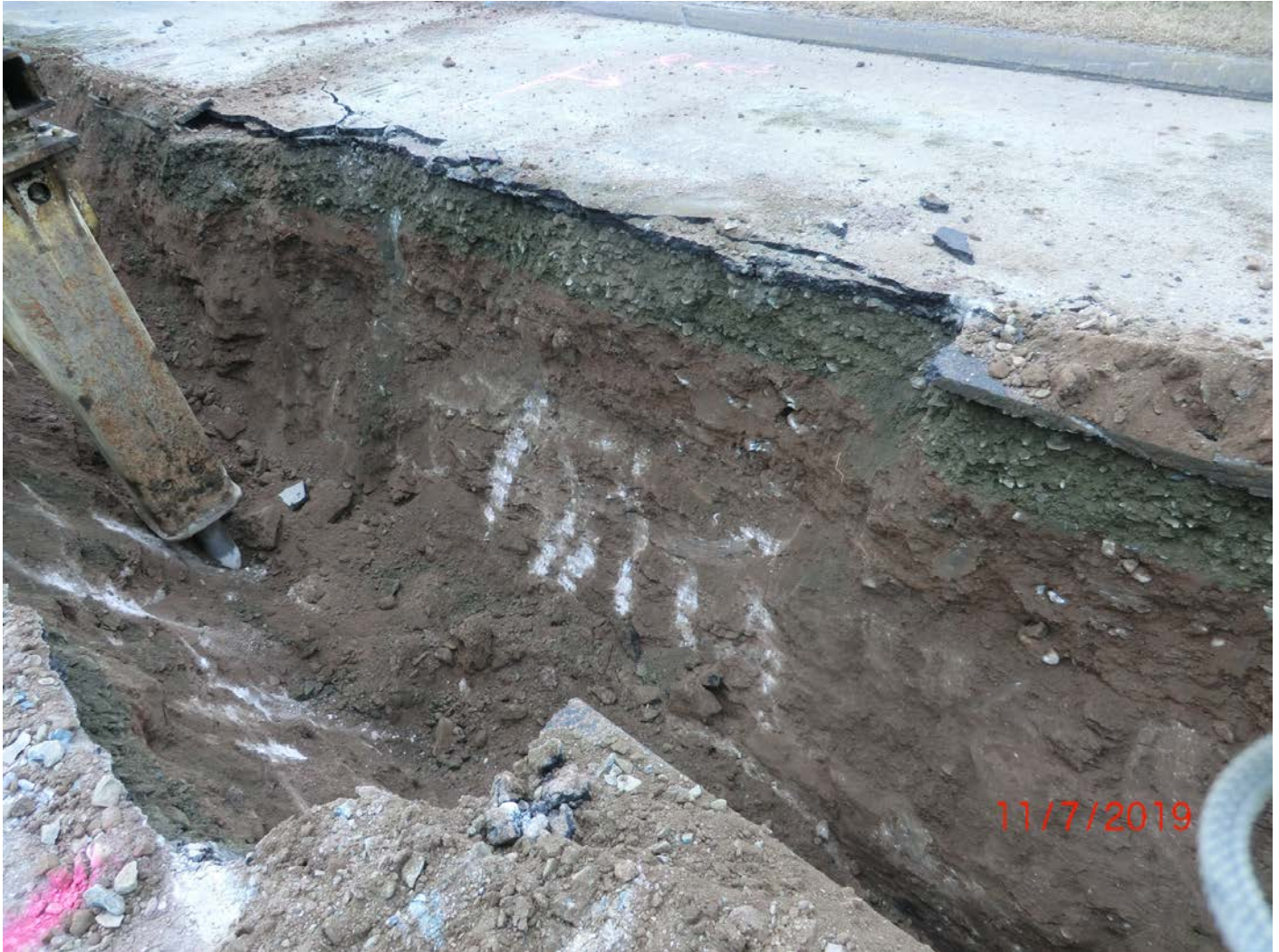
Figure 10 – Facing southwest, bedrock encountered at shallow depth along todays run. Scraped trench sides show the extent of bedrock, which starts just under the red unit.
